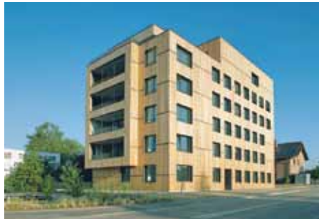
Six-storey timber construction in Steinhausen, made from prefabricated elements. (Source: Renggli AG)
