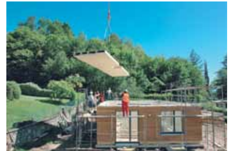
More and more frequently, timber constructions are being built from prefabricated elements. A high quality joining technique is essential. (Source: Renggli AG)
